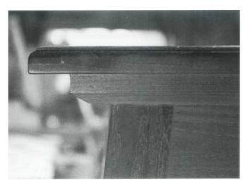
2 Screws passing up through this moulding into the top and passing through the apron into the moulding hold the top to the base.
