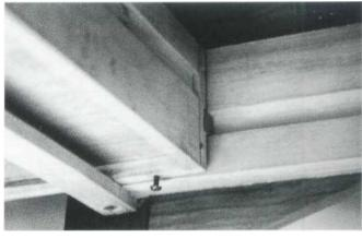
The drawer can be seen sliding in the groove ploughed in the drawer guide. When the screw turned into the bottom of the drawer side strikes the stop strip, the drawer is prevented from being pulled completely from the table.
