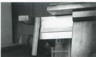
**3** Fasten the drawer runner, which slides in the groove ploughed in the drawer guides, to the drawer via several wood screws passing through the drawer side into the slide. Note the shim between the drawer front and the apron. This causes the apron to be canted at the same angle as the table's legs. Note also the spline set into the end grain of the apron. This prevents the corners of the apron from breaking off because of the grain runout on the apron's triangular tips.
