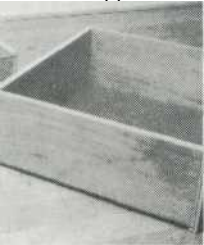
Nail Q to R using 1" brads. Slide hard-board T into groove in Q and nail. Follow the same procedure for the large drawer.
