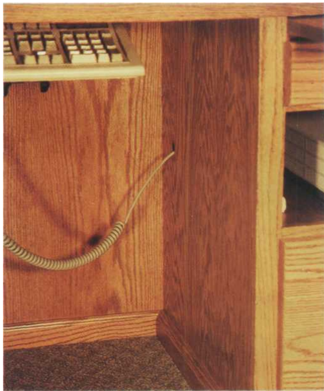
9 This detailed photo shows the hole cut in the drawer section's left bulkhead for the keyboard wire.
