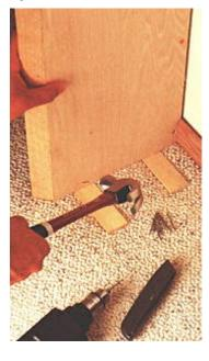
13. Drill pilot holes, then toenail the cabinet to the floor at shim locations, using 2" finish nails. Score the shims with a util Copyright 2004 Martina Auetions
