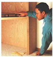
**12.** Shim below the side panels, if necessary, to bring the cabinet to level.
