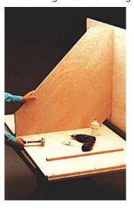
4. Measure and cut the desktop, then apply glue to the tops of the desktop cleats mounted on the back panels. Set the desktop on the cleats, then attach \$41
