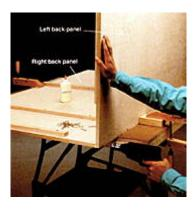
2. Clamp right back panel (38 1/4" wide) to your workbench, then apply glue to back edge. Butt left panel (39") against glued edge, and hold in place with clamps. Join back panels by drilling pilot holes and driving 2" screws through butt joint.
