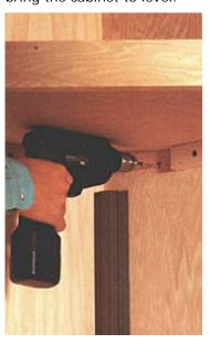
14. Attach the cabinet to the wall with 3" screws driven through the back panels and into wall studs.Drive screws just behind or below shelf cleats to keep them out of sight.
