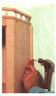
**15.** Measure and cut base shoe molding to cover the gap between the cabinet and the walls and floor, using 1 1/2" finish nails. **TIP:** To protect wall from oil or paint, insert plastic between molding and wall as you attach the molding.
