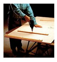
1. Measure and cut back panels (left panel overlaps right panel, so it is 3/4" wider than right panel). Cut and attach 1  $\times$  2 cleats. Drill counterbored pilot holes in cleats, then attach cleats with glue and 1 1/4" screws.
