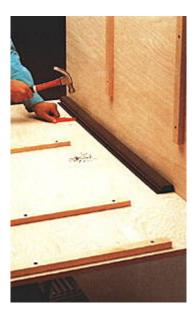
3. Attach a plastic wire organizer to one back panel edge, next to the corner joint using 1" wire nails. (Skip Copyright 2004 Martian Auctions
