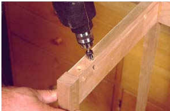
Photo 17- Now you do need the countersink. Use it to expand the top 1/4" of the hole in the rail to give the screw room to move as the tabletop changes dimension with changes in humidity.
