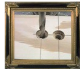
Drilling the Bolt Hole
