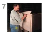
The last step on the crown is to attach the cap to the crown and cabinet. Notice the glue blocks behind the crown moulding to support the crown and add stability.
