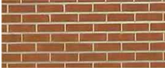
Stretcher bond is the commonest bond used today and the least interesting in appearance. It can be made more interesting by laying a course of different coloured bricks or to lay such bricks to form a pattern on a wall.
