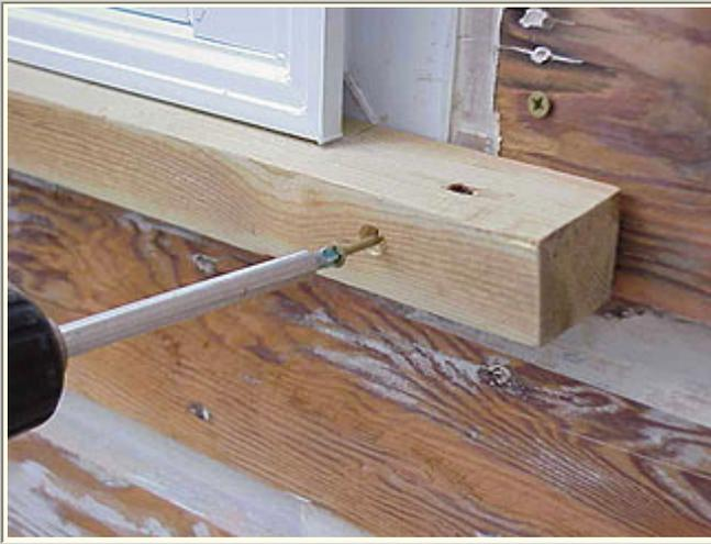
I made a **window sill** from treated pine. This was simply a piece of knot-free 2x4 that I ripped at a 10 degree angle on my table saw.
