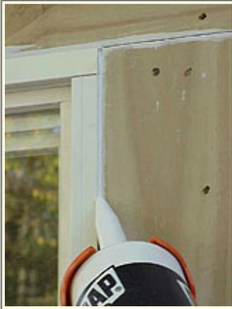
I applied caulking all over the place, especially between the window frame and the wood casing.
