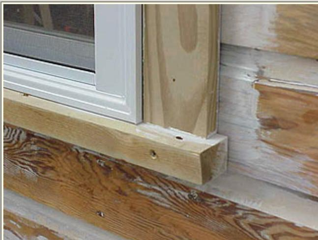
I installed 1x4 treated pine on the sides. The lower edge of this piece was cut at the same 10 degree angle, so it mated with the sloped sill.
