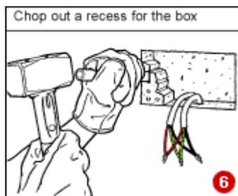
**Step 4:** Use a bolster or cold chisel to chop out a neat rectangular recess for the new box. Drill fixing holes and fit wall plugs.
