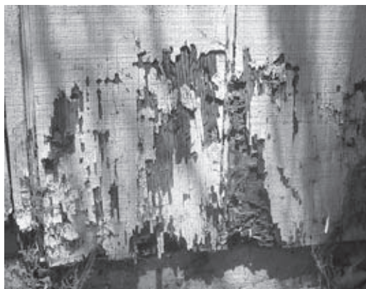
Termite-damaged wood
