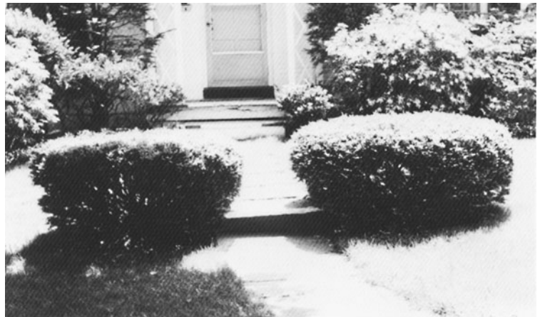
Fig. 4-1. A single step in the middle of a path is a potential hazard. The shrubs on both sides of this path call attention to the step. However, there should also be an outdoor light in the area.
