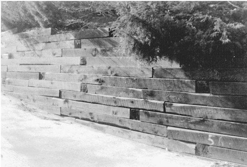
Fig. 6-12. Timber retaining wall. Note the end sections, indicating tiebacks used for anchoring the wall.
