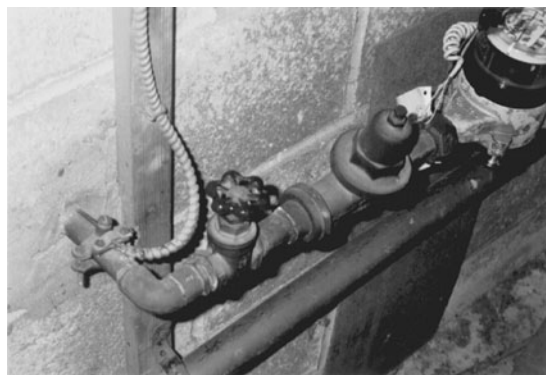
Fig. 12-8. Ground wire clamped to inlet water pipe.
