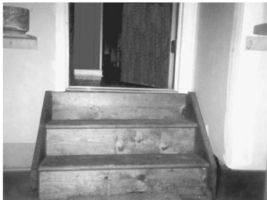
Fig. 7-1. Steps connecting the garage floor slab to the adjacent living area, which is at a higher level.
