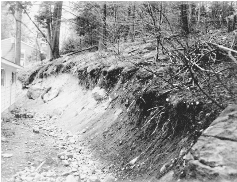
Fig. 6-4. House located on the cutout side of a hill. The building site requires special provisions to minimize erosion and drainage problems.
