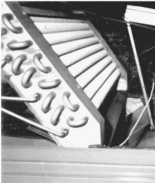
Fig. 17-4. Evaporator (cooling) coil mounted in furnace plenum.
