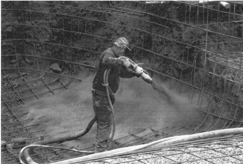
Fig. 18-1. Gunite being sprayed around reinforcing rods for a concrete swimming pool.
