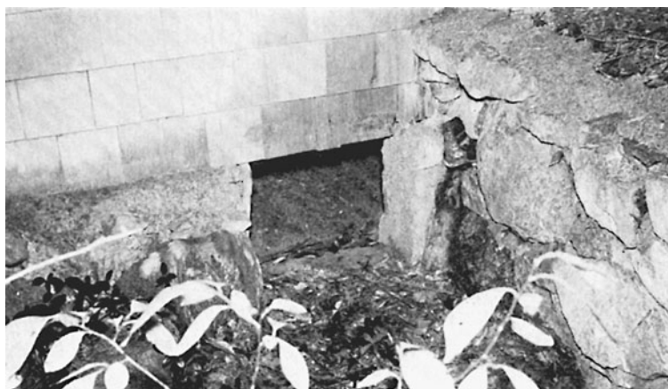
Fig. 11-16. Access hatch to crawl area.
