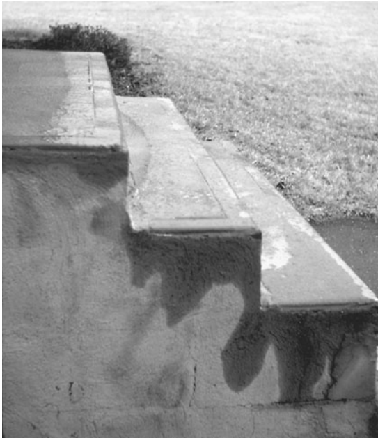
Fig. 4-2. Handrail is needed for steps, especially when they could be covered with ice.
