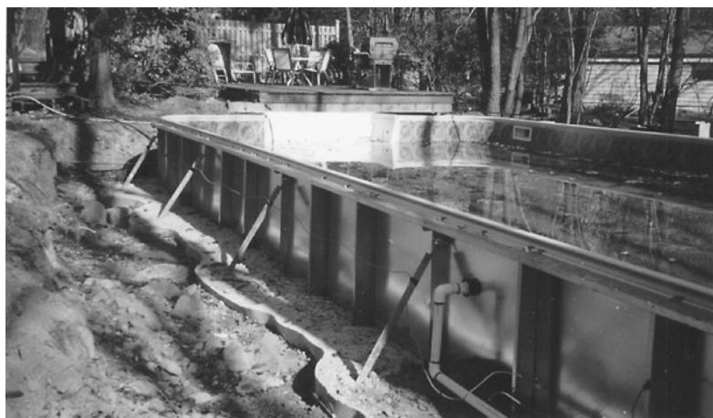
Fig. 18-3. Steel bracing for the shell of a vinyl-lined pool.
