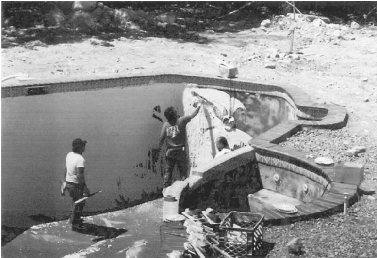
Fig. 18-2. Plaster finish being applied to a concrete pool.
