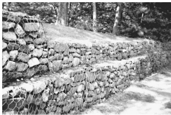
Fig. 6-10. Gabion retaining wall.
