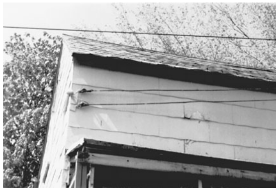
Fig. 12-1. Two-wire inlet service provides 110 volts.
