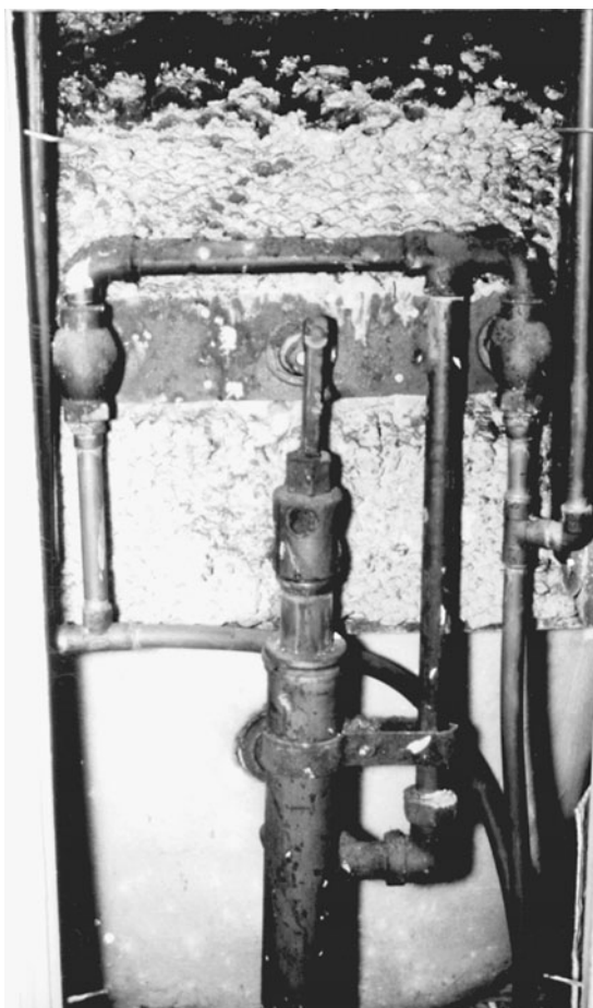
Fig. 13-7. Wall hatch in hallway provides access to pipes for bathtub.
