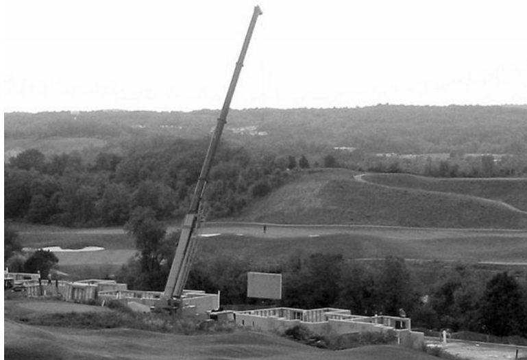
Fig. 11-3. Installing precast concrete “Superior Walls.”
