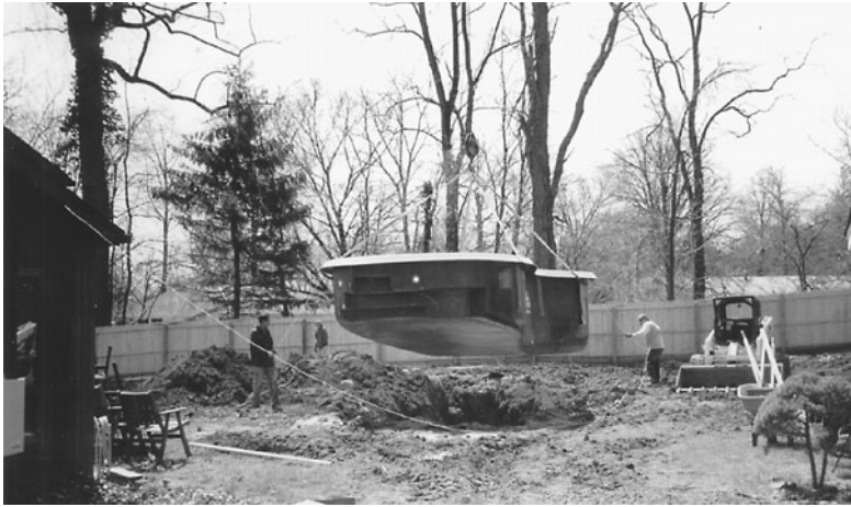
Fig. 18-4. Preformed fiberglass pool shell being installed in excavated area.
