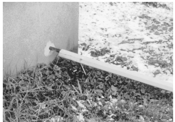
Fig. 6-8. Sump pump discharge pipes. Left—The pipe terminates just beyond the foundation wall. Right—The discharge pipe has been extended so that effluent discharges away from the foundation.
