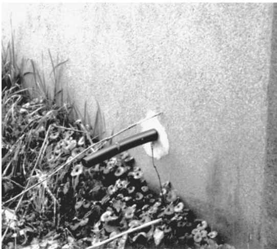
Fig. 6-8. Sump pump discharge pipes. Left—The pipe terminates just beyond the foundation wall. Right—The discharge pipe has been extended so that effluent discharges away from the foundation.
