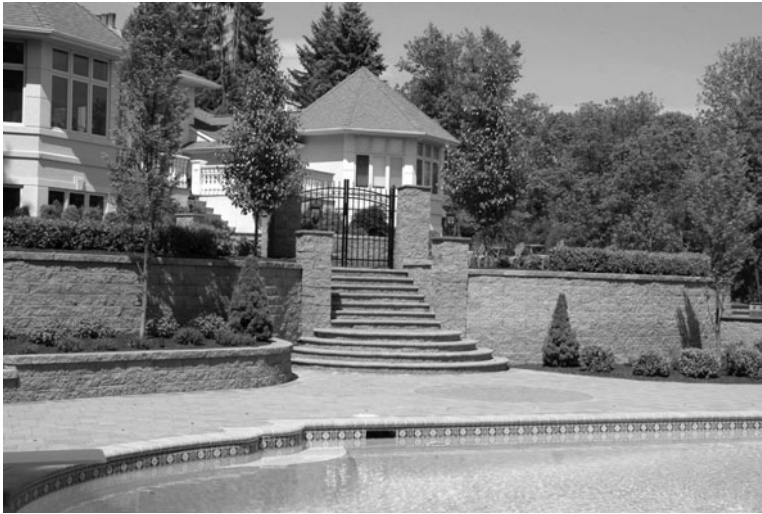
Fig. 6-14. Concrete block retaining wall.
