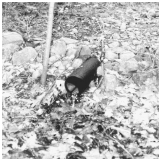
Fig. 6-9. Free-flowing outlet of curtain drain. Note water discharging from pipe.
