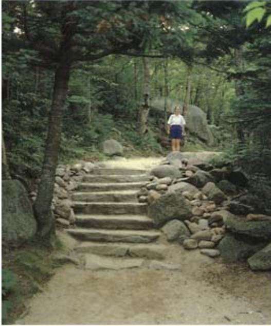
28 A well-designed and well-constructed set of stone steps, which are blended into the boulder-strewn landform. Mother Walker Falls State Park, Maine, USA.
