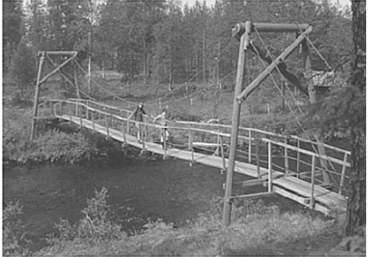
*An example of a fairly basic suspension bridge over a river in Finnish Lapland. The main cables should be tightened to prevent the sag in the middle and to reduce the swing and bounce experienced when crossing the bridge.*
