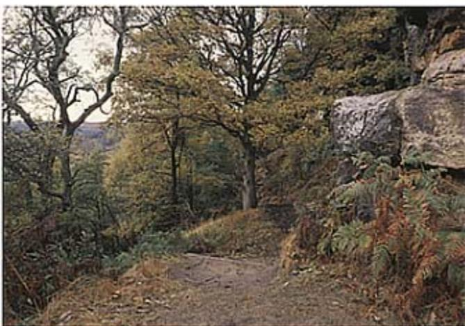
27 A good example of a path cut in a side slope on mineral soil. Re-vegetation of the
