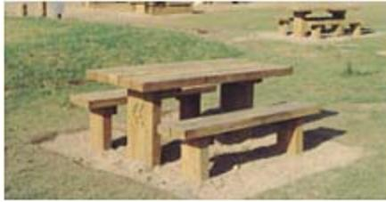
19 This is a well-designed example from Britain's Forest Enterprise. It has the right proportions, and is placed level. The unit has been set into the ground so that there are no obstructions to visitors' legs or feet. An area around the unit has been laid with gravel to prevent wear and tear of the surface. Where there is easy access for people with disabilities the table-top can be extended so that a wheelchair can be set at it. Beechenhurst, Forest of Dean, Gloucestershire, England.
