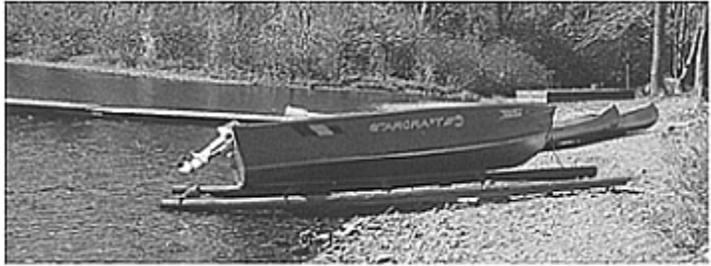
*A simple, small boat-launching ramp, which uses rollers on a timber frame to ease the task of hauling a dinghy from the lake. Baxter State Park, Maine, USA.*
