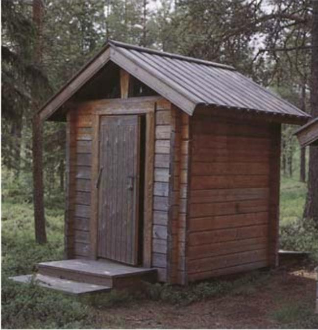
17 This Swedish example is an excellent composting toilet. The sawn log construction is sturdy. It uses traditional overlapping boards for the roof. Windows in the gable give adequate light and privacy.
