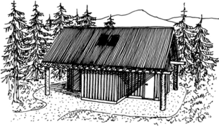
*A toilet building designed for a forest landscape. Coarse textures of cladding and roof, exposed beam ends and the use of large dimension timbers work rather well.*
