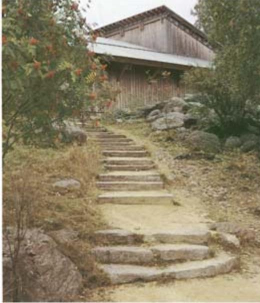
5 A more recent example from Germany uses natural stone, gravel and weathered rough sawn timber, which work together and fit their surroundings. Simplicity and good attention to the detail of construction make this a timeless solution.
