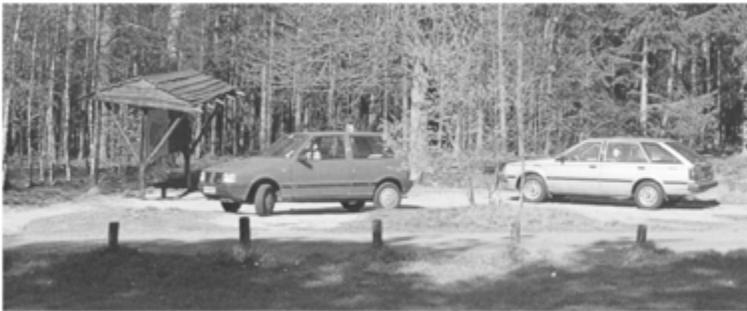
*Log posts set into the ground work well, especially in wooded settings. Near Hilversum, Holland.*
