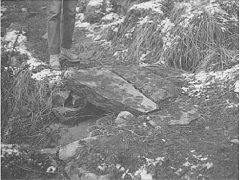
*An example of a box culvert made from local stone and covered in large flat slabs. This is an attractive and durable solution. Glen Affric, Scotland.*
