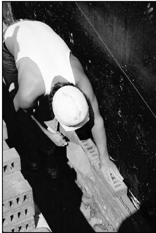
Using brick and mortar, Andy builds a wall according to a blueprint.
