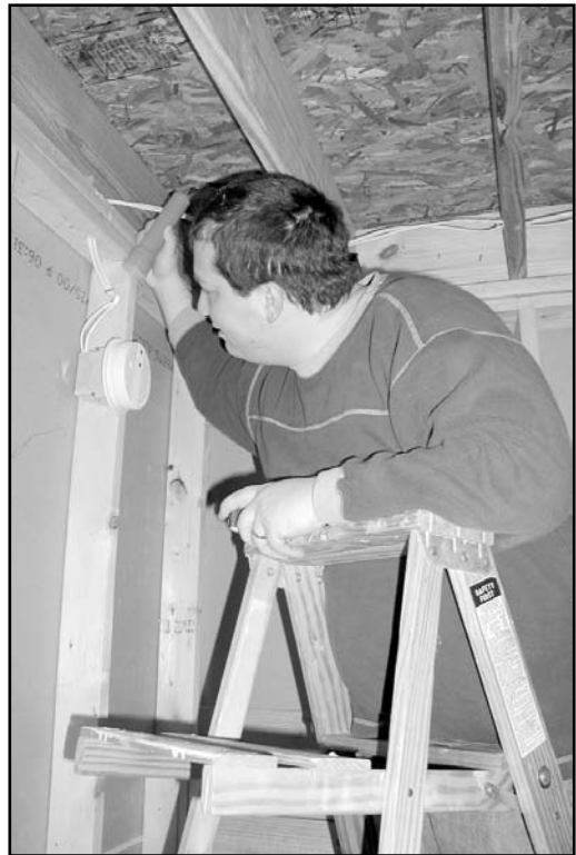
A home inspector checks wiring, plumbing, and other structural components of a house.
