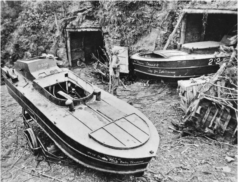
A Marine stands guard near Shinyo found on Aka Jima, Kerama Retto. These Shinyo were hidden in caves and then transported to the water on trailers. The trailer can be seen under the nearest Shinyo . Official USMC photograph.
