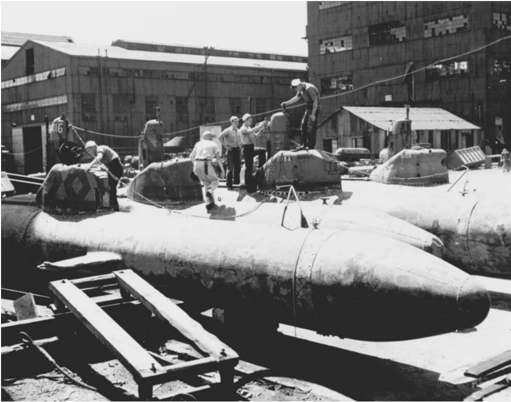
American sailors inspect a Kairyu submarine at Yokosuka Naval Yard, 11 September 1945. These subs were fitted with an explosive warhead. NARA 80G 338383.
