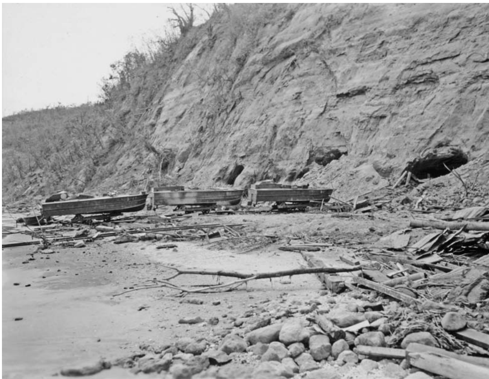
Three Imperial Navy Shinyo suicide boats are shown on tracks leading from their cave to the water on Corregidor. A series of caves may be seen in the cliff side. This made it difficult to eradicate the boats with air or naval attack, but left them vulnerable to disaster if one caught fire in the tunnel. This photograph was taken on 27 February 1945. NARA 111-SC-263697.
