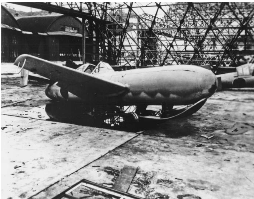
An Oka unpowered trainer shown after the war. Water ballast was used in place of the heavy explosive charge and jettisoned just prior to landing. The skid was used in place of wheels. NARA 80G 193349.
