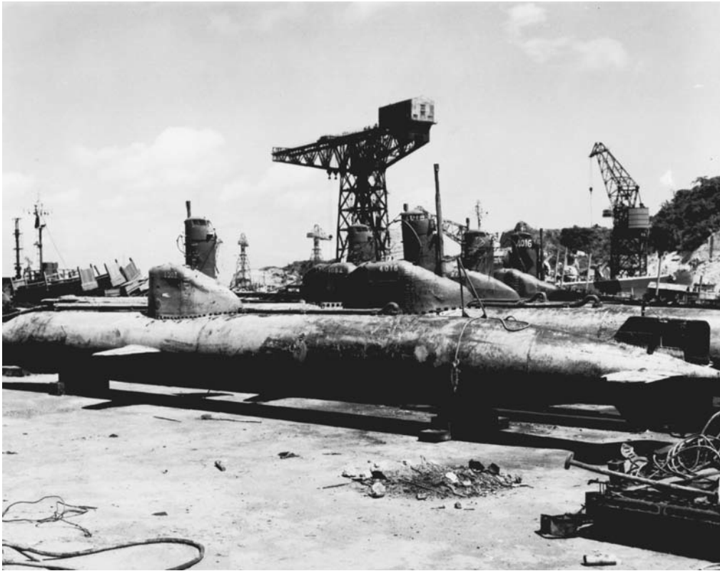
Kairyu submarines at Yokosuka shipyard on 11 September 1945. Subs numbered 4018 and 4016 can be identified as training subs because they have two periscopes and a longer sail. NARA 80G 338384.
