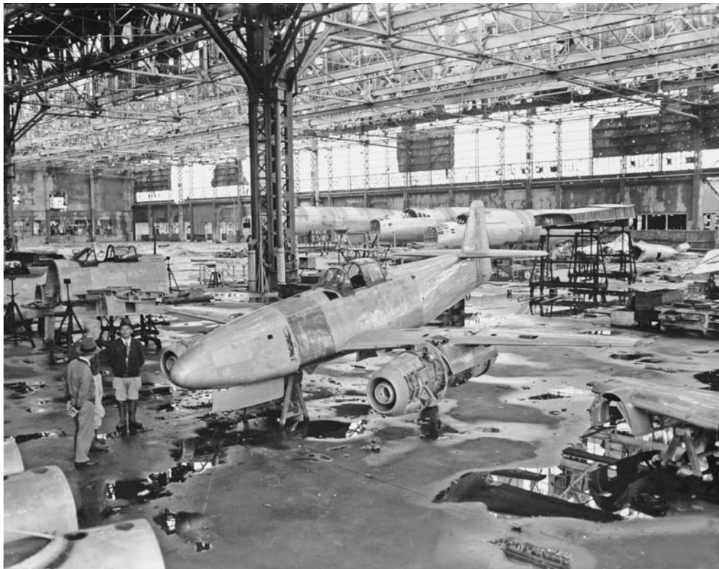
This Japanese twin-engine jet, the Nakajima Kikka (Orange Blossom), is shown under construction at the Nakajima factory on Honshu on 6 October 1945. NARA 111-SC-225102.
