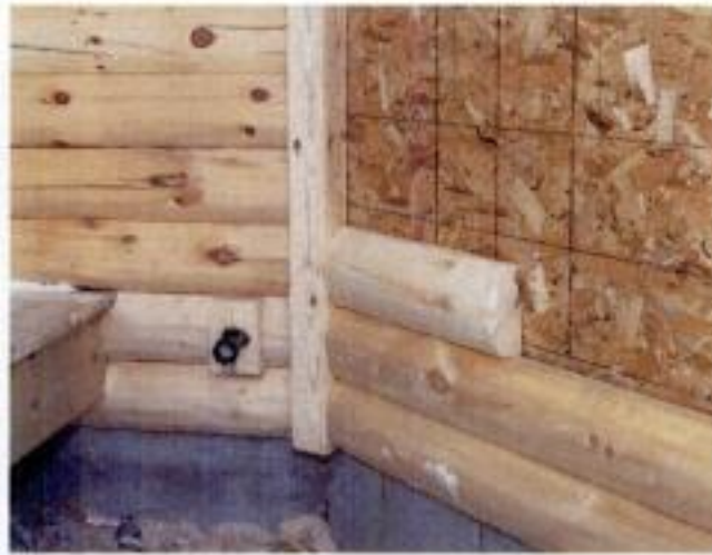
The full-log system met the half-log system in several places, including this corner between the front porch and the garage (above left). The half-log system so closely replicates the look of the full-log system it's difficult to tell where one ends and the other begins. This shot of a partially-covered garage wall (above middle) is a good example. A close-up look at another corner (above right) reveals how closely the half-log system matches the full log system, even duplicating the butt and pass corner system.
