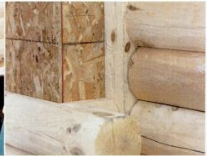
The full-log system met the half-log system in several places, including this corner between the front porch and the garage (above left). The half-log system so closely replicates the look of the full-log system it's difficult to tell where one ends and the other begins. This shot of a partially-covered garage wall (above middle) is a good example. A close-up look at another corner (above right) reveals how closely the half-log system matches the full log system, even duplicating the butt and pass corner system.
