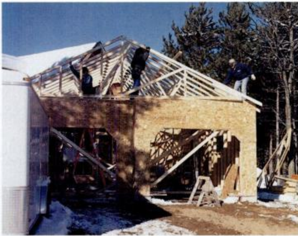
Earlier in the winter, Golden Eagle's crew installed engineered trusses from Automated Products, Inc. on the two-stall garage, which was conventionally framed.
