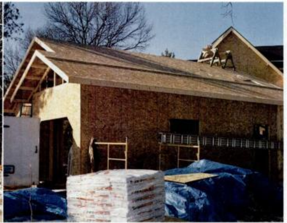
The garage was finished with oriented strand board (OSB) before half logs matching the Double Eagle's full-log system could be installed.
