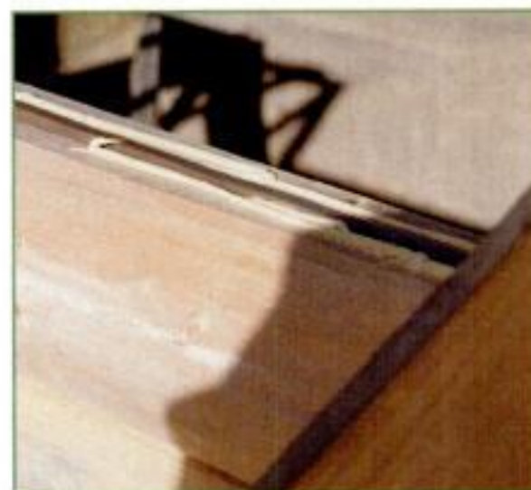
FOAM GASKET SEALANT
