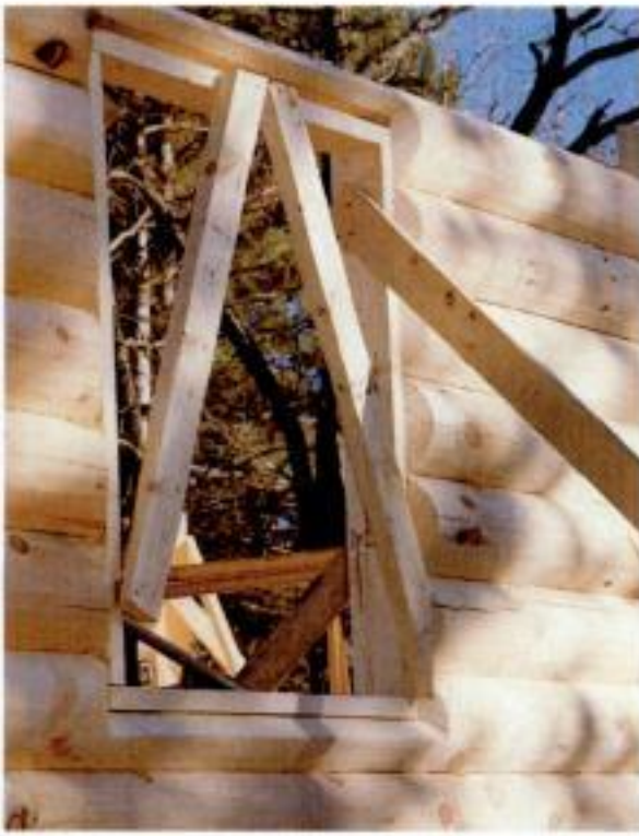
Pre-made 2x6 bucks framed the window and door openings while the logs were stacked.
