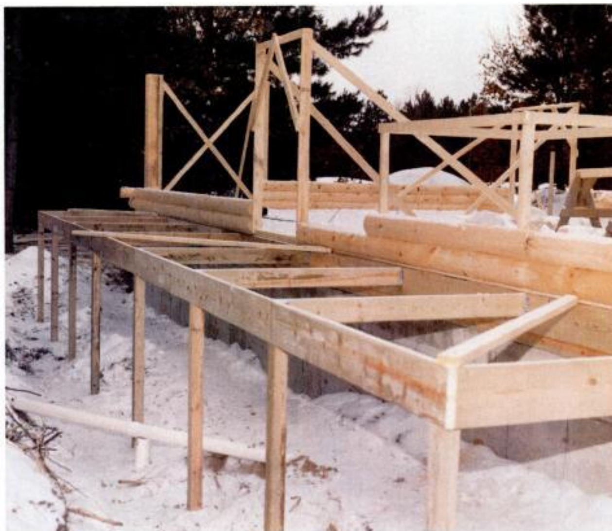
The view of what will be the front porch from the yard (above). Two full courses of logs have been laid around the perimeter.
