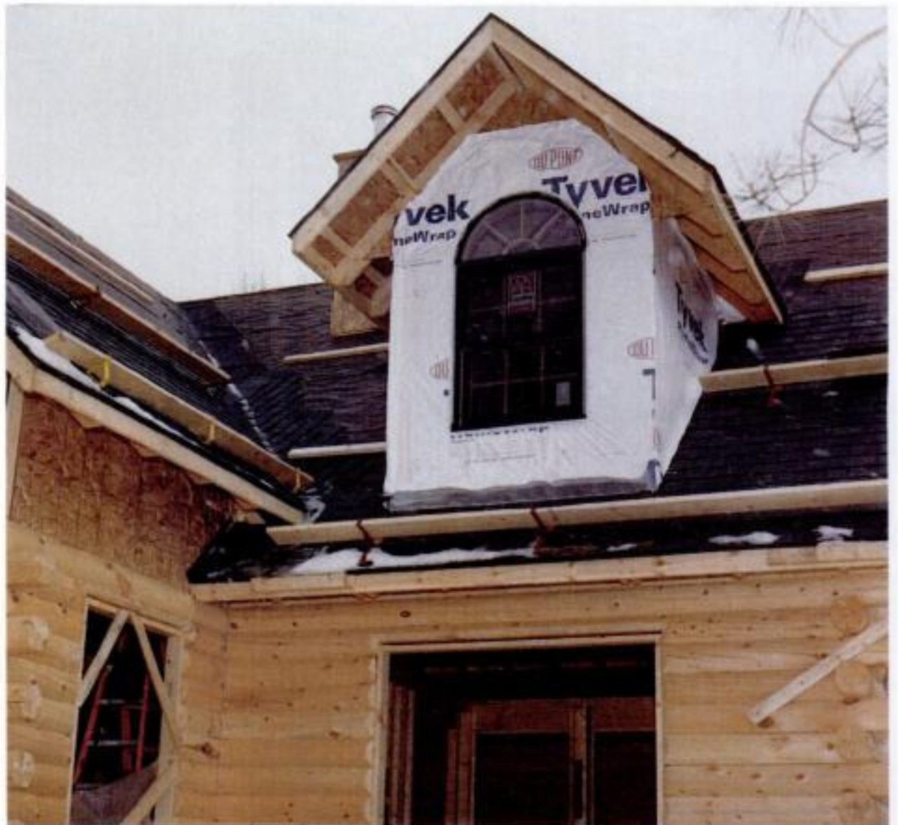
The green aluminum-clad exterior finish on the windows and doors (top) complements the shingles, soffit and fascia. The windows, shingles and half-logs were installed at the same time (above).
