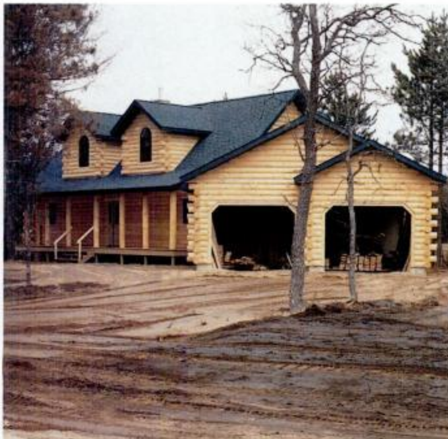
The full-log system met the half-log system in several places, including this corner between the front porch and the garage (above left). The half-log system so closely replicates the look of the full-log system it's difficult to tell where one ends and the other begins. This shot of a partially-covered garage wall (above middle) is a good example. A close-up look at another corner (above right) reveals how closely the half-log system matches the full log system, even duplicating the butt and pass corner system.
