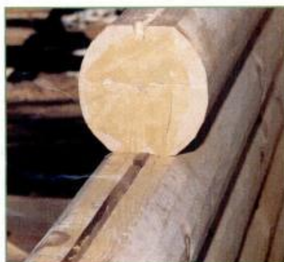
GROOVE & GASKET JOINERY
