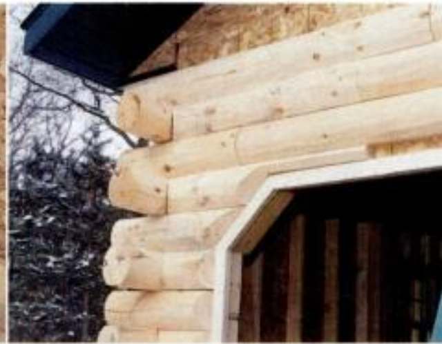
The full-log system met the half-log system in several places, including this corner between the front porch and the garage (above left). The half-log system so closely replicates the look of the full-log system it's difficult to tell where one ends and the other begins. This shot of a partially-covered garage wall (above middle) is a good example. A close-up look at another corner (above right) reveals how closely the half-log system matches the full log system, even duplicating the butt and pass corner system.
