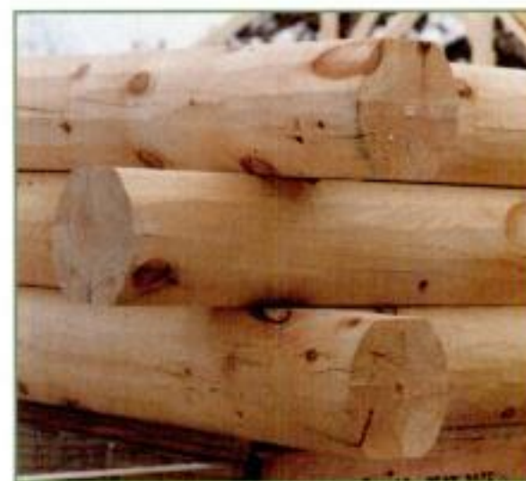
BUTT & PASS CORNER SYSTEM
