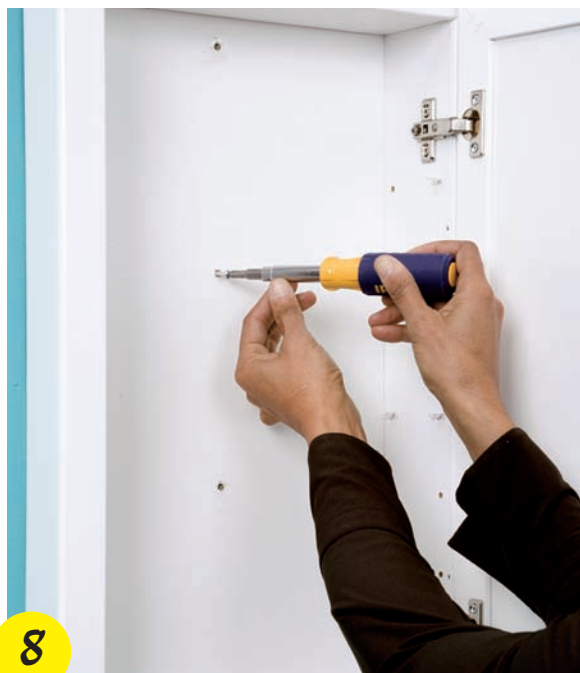
Screw the cabinet to the wall with a screwdriver.
