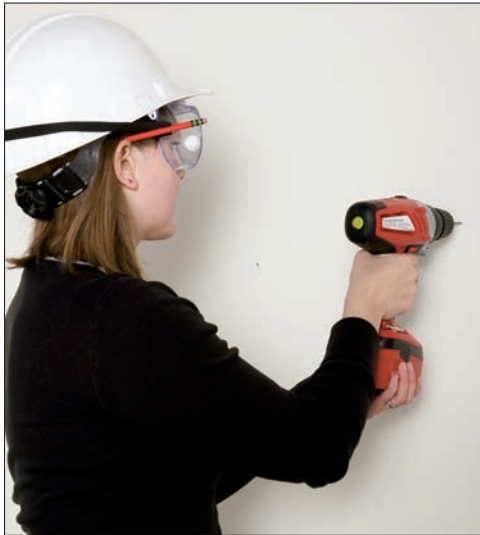
Figure 3-2: Drill your holes perpendicular to a wall by starting off at the right height.
