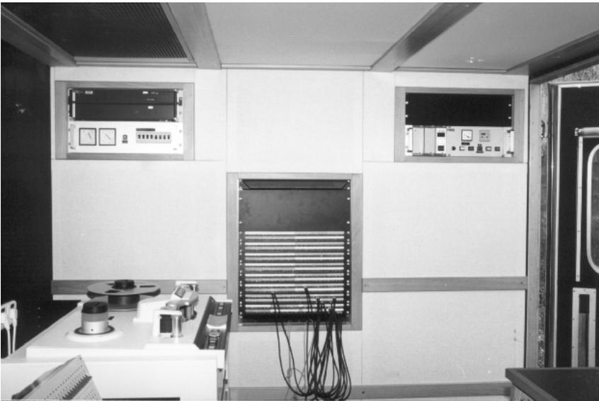
**Figure 23.8** The completed rear-wall absorber system
