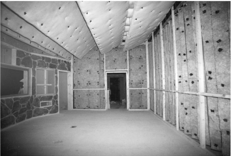
**Figure A.1.11** The completed acoustic control system at Area Master studios, Vigo, Spain; viewed from the rear, and showing the closed nature of the ceiling panels from this viewpoint. Compare this with the view in Figure A.1.12
