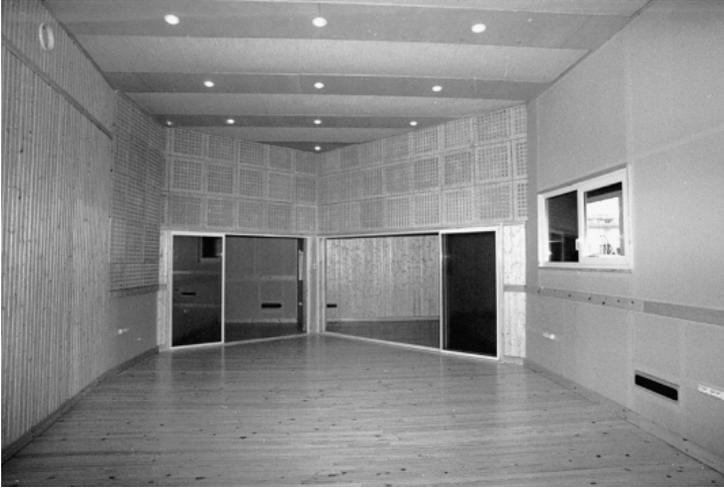
**Figure 7.1** Dobrolyot Studio, St Petersburg, Russia (1996). Note the ex-Soviet era perforated diffusers over the glass doors and on the adjacent left-hand wall. (See also on the front cover.)
