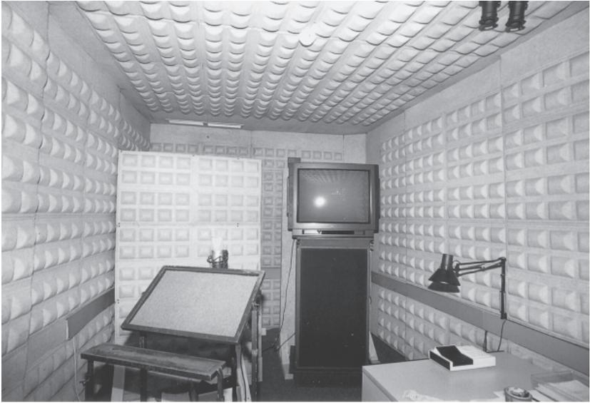
**Figure 5.24** A voice recording room constructed without the required space behind the ‘absorbent’ panels on the walls and ceiling
