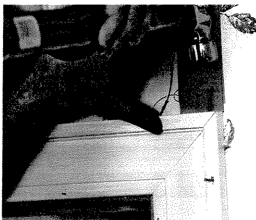
With the side casings temporarily in place, measure for your top piece.
