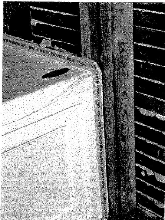
The stud closest to the tub is a nailer for wallboard. The middle stud serves as a nailer for the tub and, together with the third stud, for the shower door.
