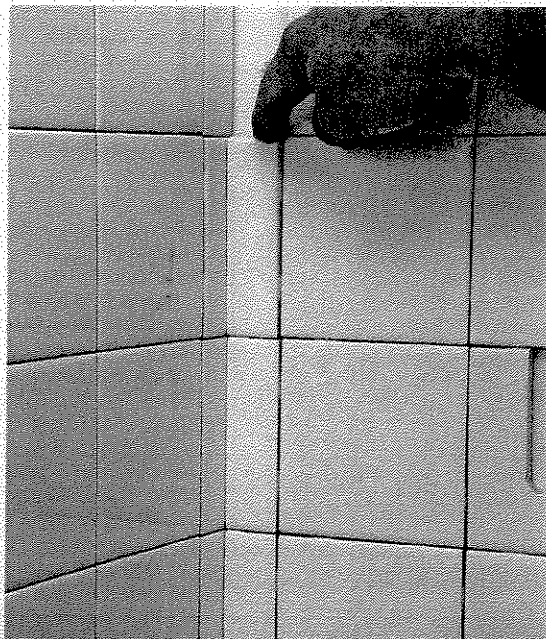
If the piece is tight, don't force it into the corner; cut another one instead.
