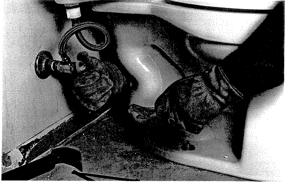
Make sure the water does indeed turn off completely; if it doesn't, turn off the main water supply and change the shut-off valve to the toilet.
