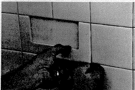
Here tiles need to be cut to fill in around the soap dish. It looks better if the tiles are cut equally.
