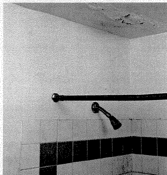
With a leak like this, it's just a matter of time before the ceiling falls down due to the weight of the water absorbed by the wallboard.
