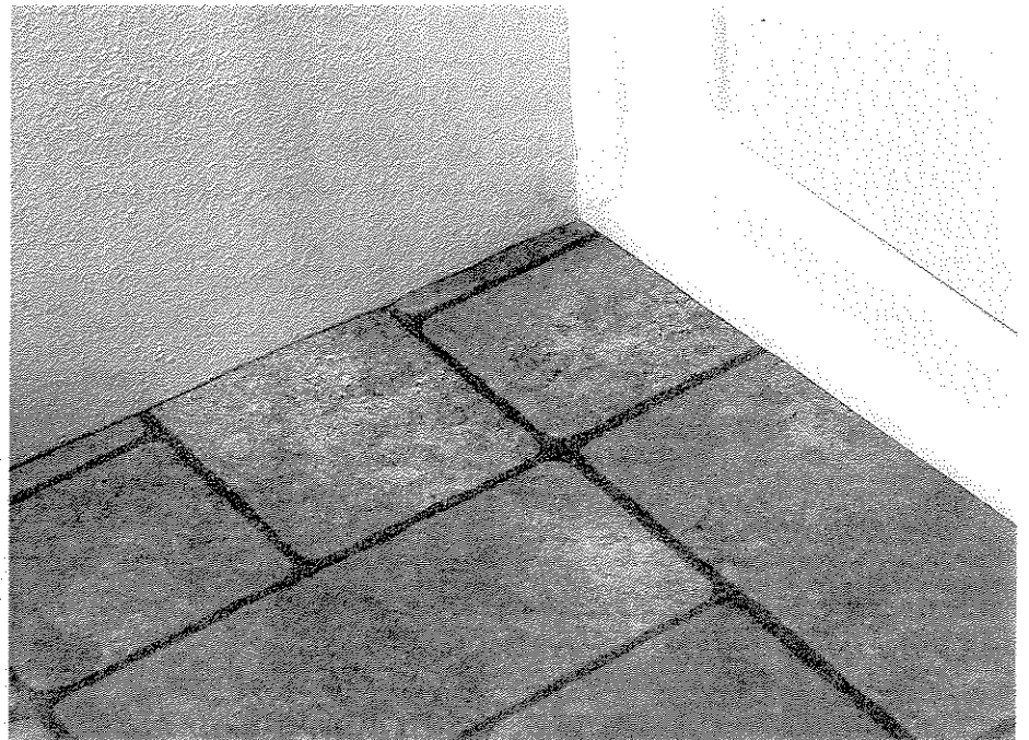
Rubber base molding will cover the grout lines close to the wall.
