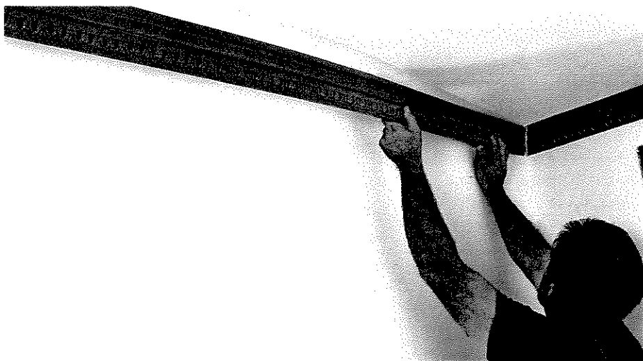
Because urethane molding expands and contracts, I recommend that you add 1/4 in. to every 10 ft. and spring the longer moldings into place.
