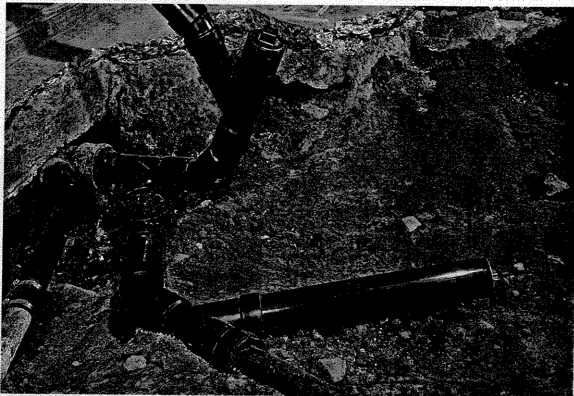
This very accessible 3-in. ABS cleanout was installed after replacing all the 4-in. cast-iron pipe to the upstairs bathroom. The drainpipes shown will serve our new bath-laundry in the basement.
