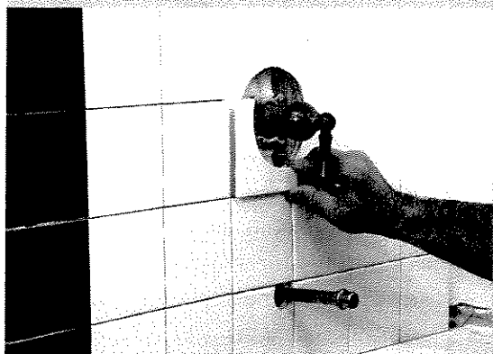
Cut the tile carefully around the plumbing fittings for a professional finish.
