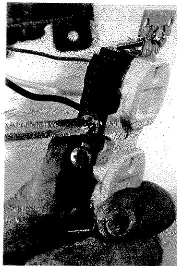
Loop the wire clockwise around the terminal screw so that the wire locks tightly against the terminal for a secure installation.
