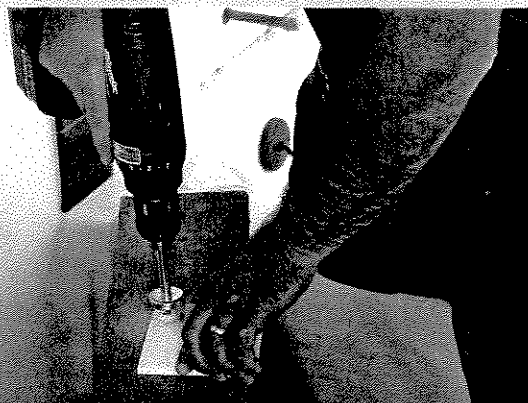
A carbide ceramic hole saw cuts a clean hole. Drill from the finish side; wear eye protection.
