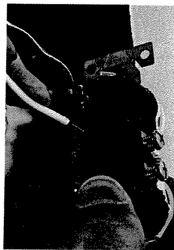
Wire, which is pushed into the wire well with these push-in outlets, is automatically clamped by spring action to ensure good electrical connection.
