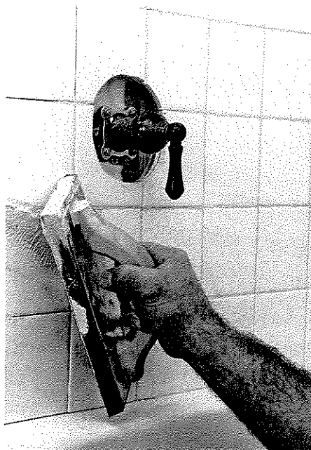
Work grout into all joints using a rubber grout float.
