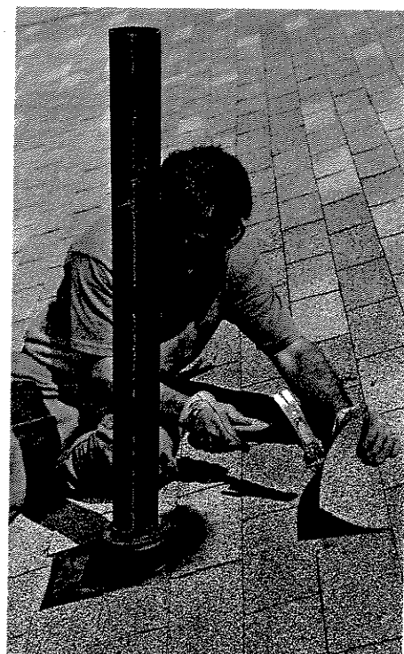
With the flashing in place, I can reinstall the 3-tab roofing material, trimming it around the flashing collar. Now the vent pipe needs to be cut for height.
