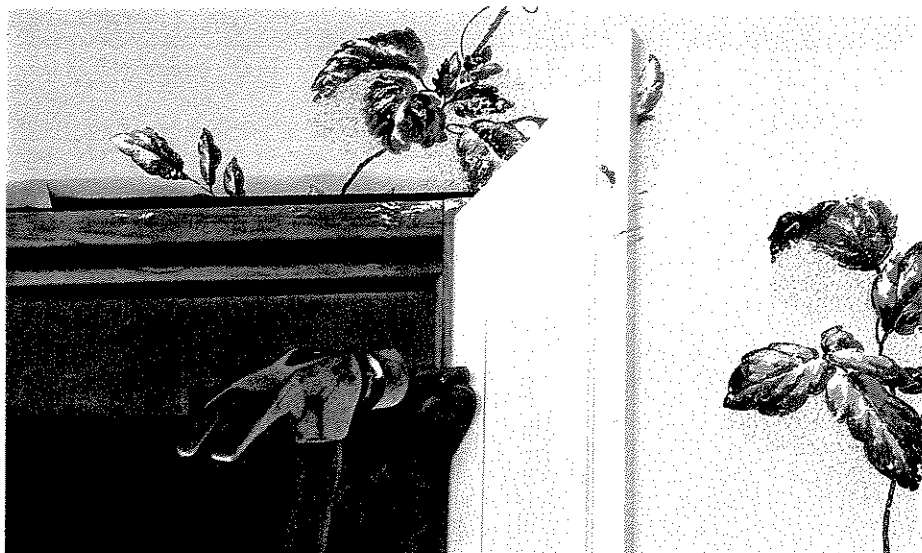
Drive nails partially until you trial fit the next piece of casing.
