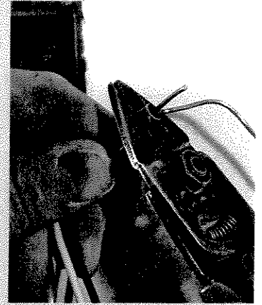
Slide the ground crimp connector over the wire and hold it long enough to get the crimping tool around it. Don't let go of the ground wires—then squeeze the crimping tool.
