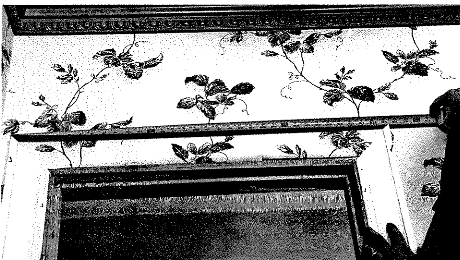
With the side casings temporarily in place, measure for your top piece.
