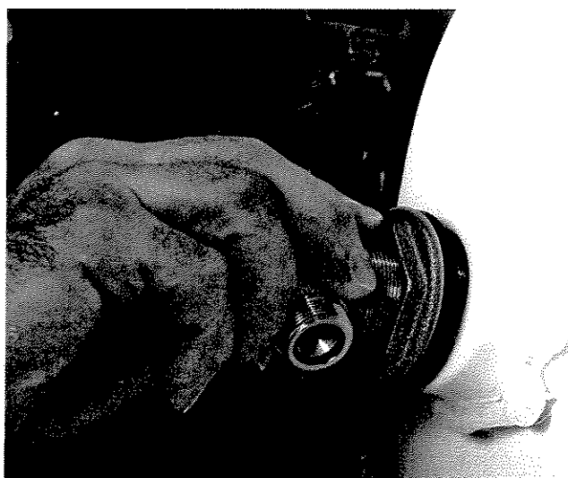
Be sure to fill the perimeter cavity of the plastic bottom plate with plumber's putty.
