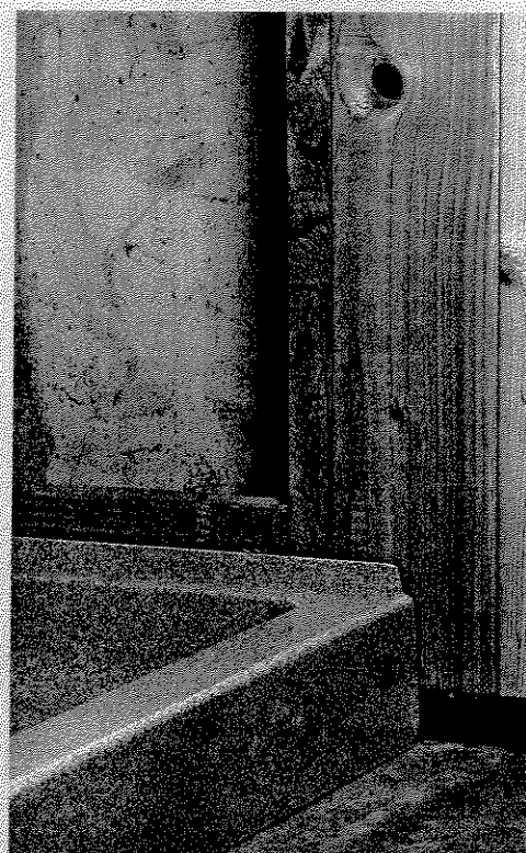
A backer board nailed to the partition provides framing for the shower pan.
