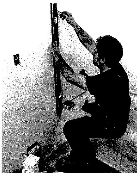
A vertical pencil line guides tile placement on the sidewall.
