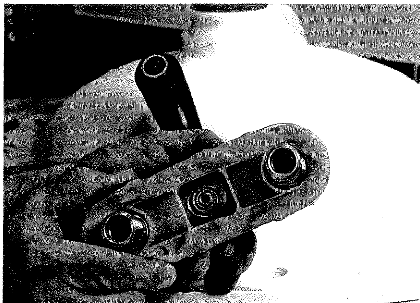
Be sure to fill the perimeter cavity of the plastic bottom plate with plumber's putty.
