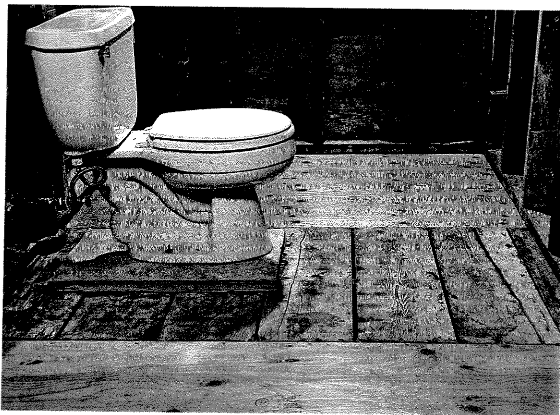
Most of the subfloor has been replaced; the toilet area is the only section remaining. The main soil pipe will be moved once the cast-iron pipe is replaced with one made of plastic called ABS (acrylonitrile butadiene styrene).
