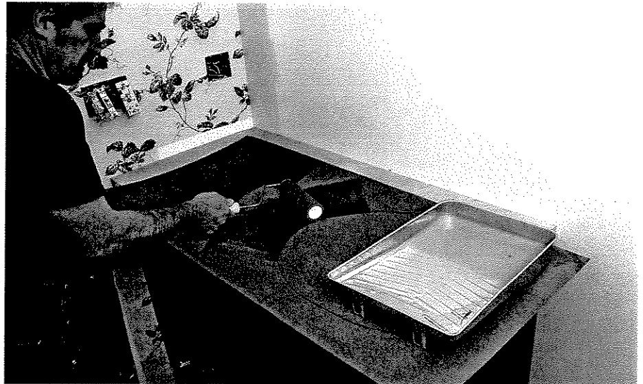
Make sure glue completely covers all but the sink-cutout area.
