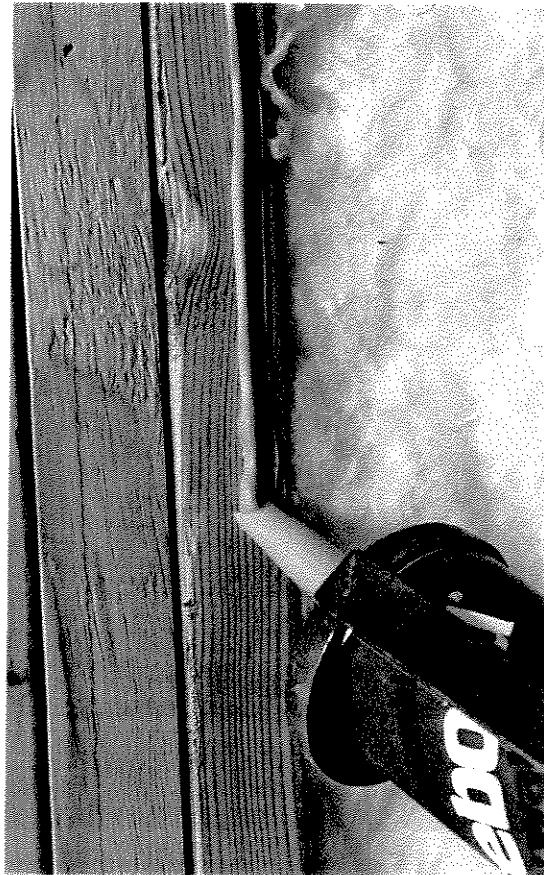
Cutting the tip of the tube properly will help you smoothly apply the correct amount of adhesive to studs.
