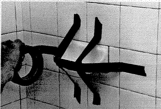
Secure the soap dish for at least 24 hours using blue painters' masking tape.
