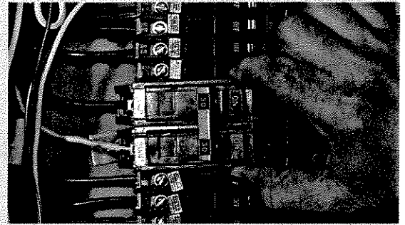
Use a double-pole breaker with 240-v circuits.
