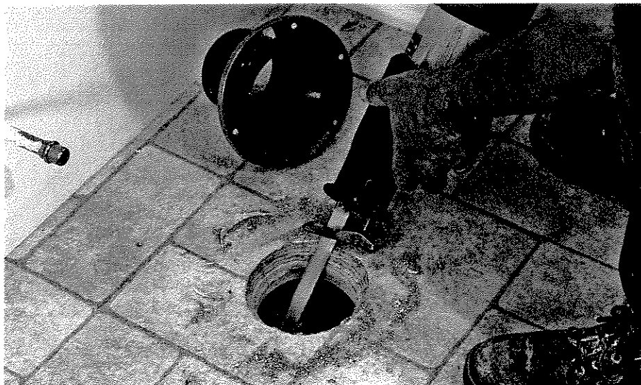
When beveling the hole to match the bevel around the bottom side of the flange, use a reciprocating saw; be aware of the saw's shoe as you don't want it to damage the floor covering.
