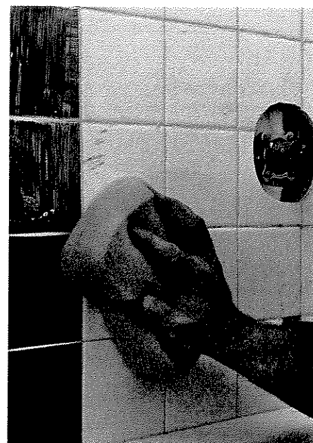
Take care not to apply too much pressure on grout joints as you clean the tiles.
