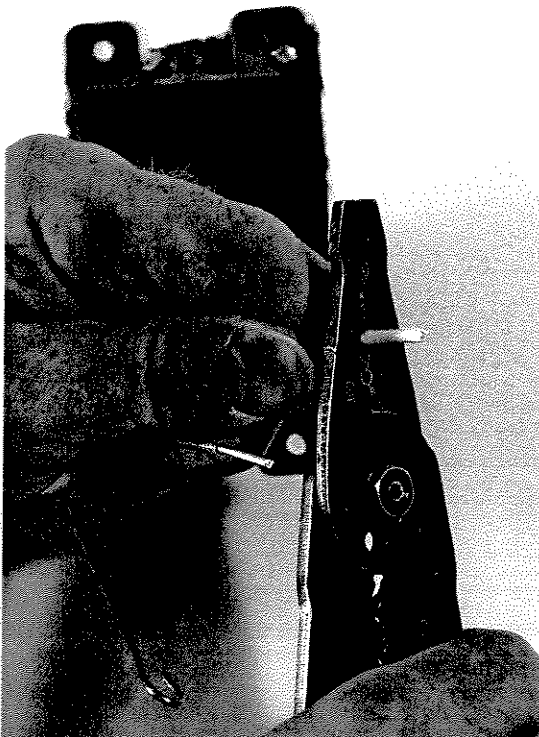
Remove \frac{1}{2} in. of insulation from the wire and attach to either the terminal screws or the push-in outlets.
