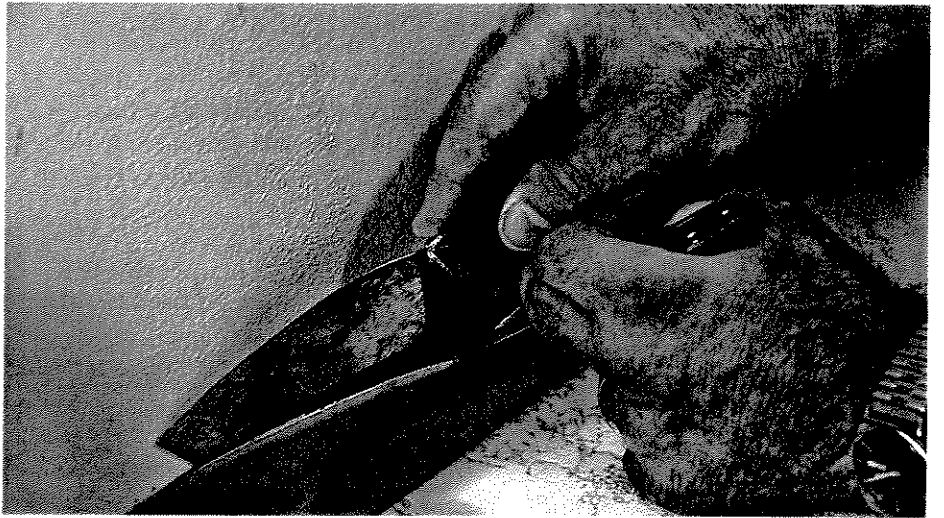
Pry rubber, vinyl, and wood base molding from the wall using a stiff putty knife.
