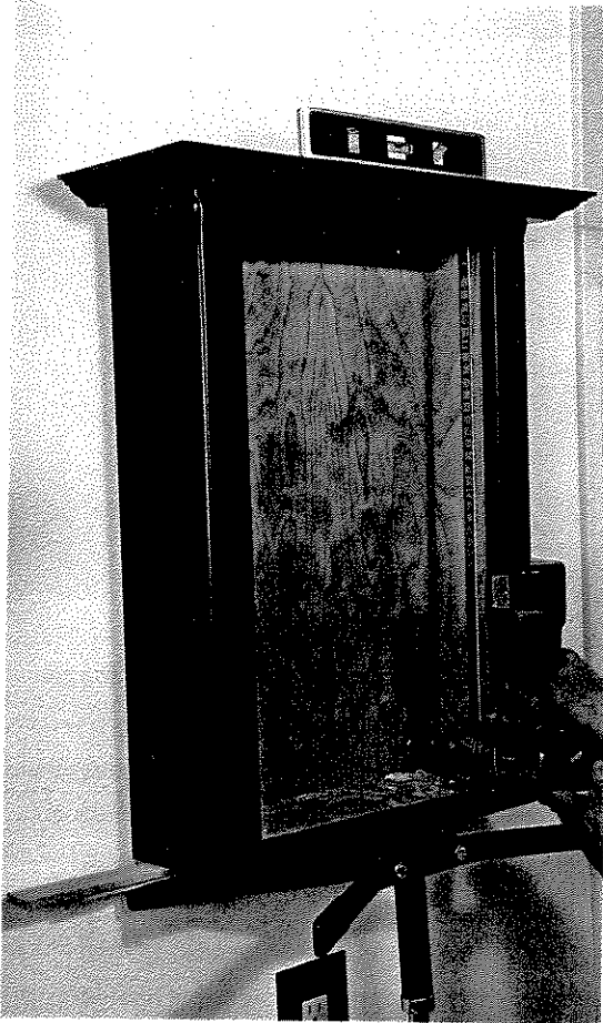
Backing installed during framing (plus a cabinet stand) made installing this custom-made cabinet easy.
