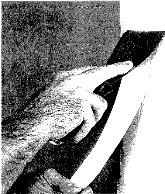
Always start at the top of vertical joints and draw the knife downward with even pressure.
