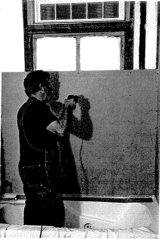
Water-resistant gypsum wallboard provides a good substrate in the tub/shower area, providing it's not installed over a vapor barrier.
