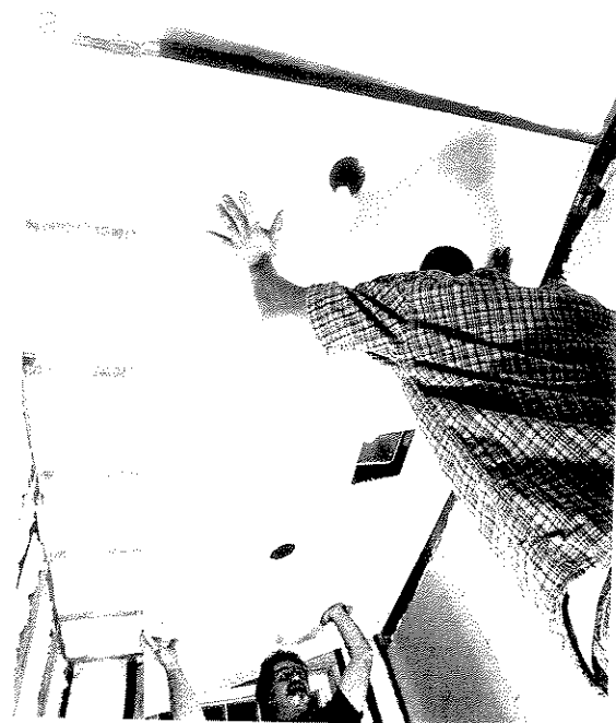
Use gypsum wallboard (not green board) for smooth and textured walls and ceilings that won't be exposed to water or long-term moisture.
