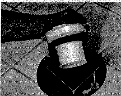
This O-ring seals tightly to block sewer gases.
