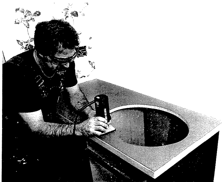
In the sink area, drill a hole in the center of the laminate that's large enough to fit the router bit comfortably. Before turning on the router, make sure the bit is not in contact with the sides of the hole.
