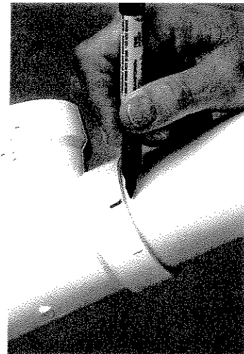
An alignment mark across each joint will assure an exact fit.
