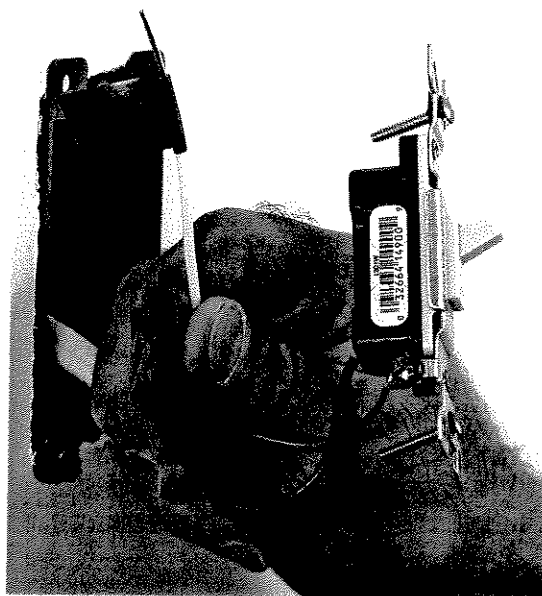
White wire has been stripped to its proper length ( \frac{1}{2} in.), and the black tape is installed just before the stripped wire.
