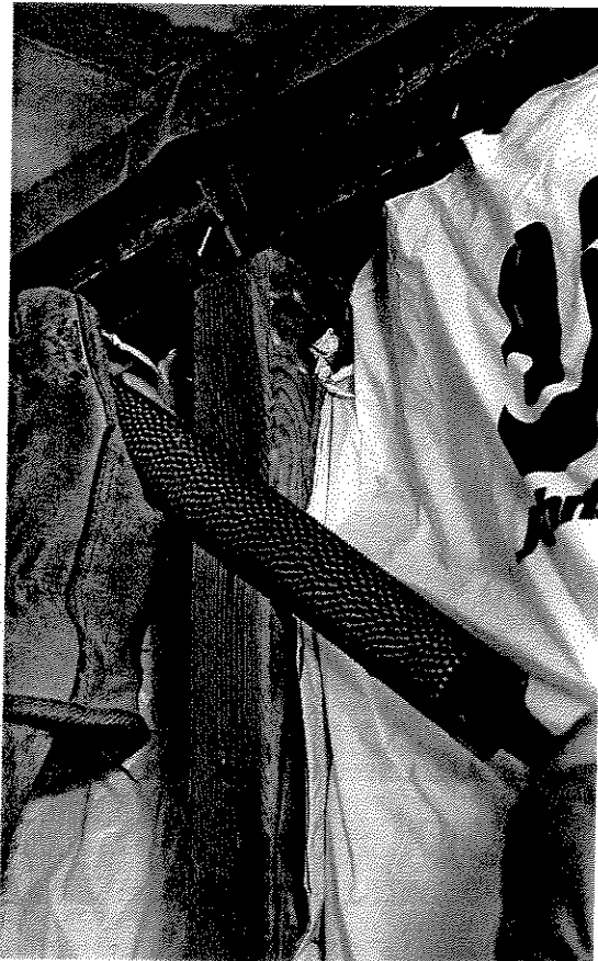
A wood rasp helps to remove a high spot on a stud.
