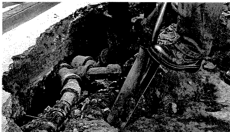
To reach the pipes, the concrete was broken up with a jackhammer and the soil removed using this drain spade.
