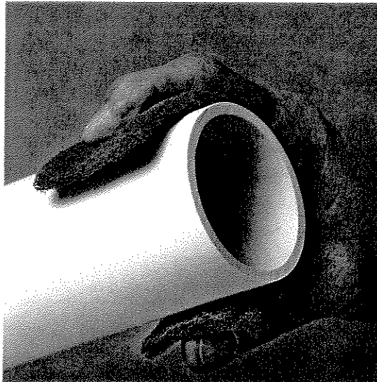
Surfaces to be glued should have a dull finish.
