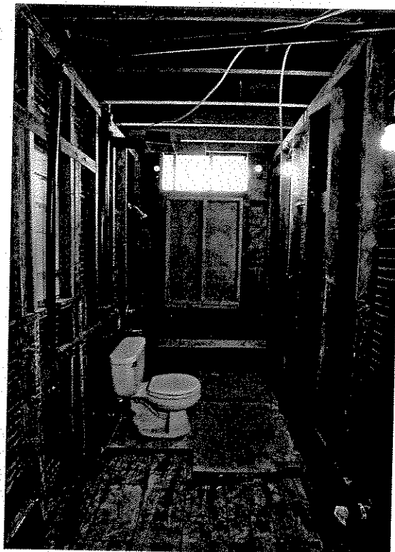
With the subfloor exposed it's easy to see water damage, which appears to have extended to boards used in construction of the foundation.
