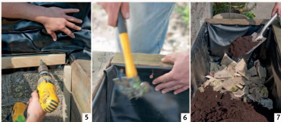
**5. Line the bed.** We used a piece of old pond liner and attached it to the wall using a wooden batten. **6. Fold the liner** to fit, then nail the edges to the frame. The liner stops moisture from soaking into the wood and keeps it in the soil. **7. Fill** the bottom 4 in (10 cm) with broken pottery and stones for drainage. Add good-quality potting mix, water it well, and start planting.
