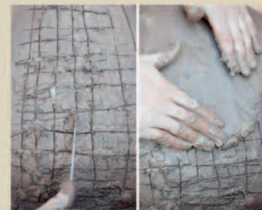
■ **Wet the surface**, then score it with a cross-hatch pattern (left). Apply more clay to the cracked area (right). Repeat if cracks appear after the oven is used.
