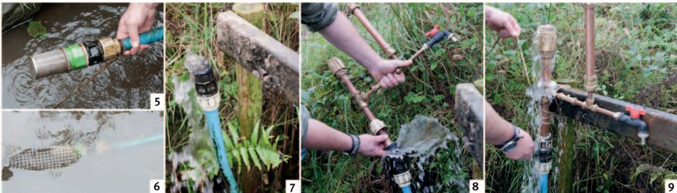
**5. Attach** a filter to the drive pipe to stop debris from clogging the system. Make sure it is submerged—we tie ours to a post under the water. **6. Add** an additional coarse mesh basket to stop larger debris from sticking to the filter. **7. Run the drive pipe** from the water source to the pump. **8. Connect the drive pipe** to the pump. Water should flow freely through the waste valve. **9. Fix the ram pump upright.** We built a frame from spare lumber and lashed the pump to it.
