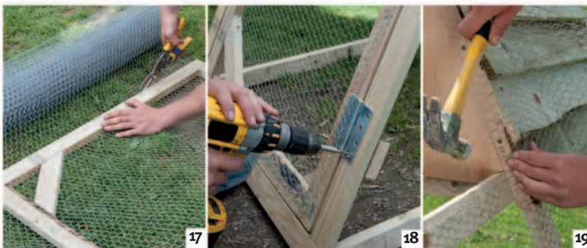
**17. Make another door** to fit one of the bottom rectangles. Strengthen the door with two corner braces at opposite ends. Attach hinges to one of the vertical sides. Cut chicken wire to size and staple it in place. **18. Screw the door hinges** in place and attach a latch to keep out predators. **19. Continue** attaching chicken wire over the whole frame, taking care not to leave any loose edges. Snip off any sharp ends. **20. Install** a drinker and feeder, and introduce your chickens!
