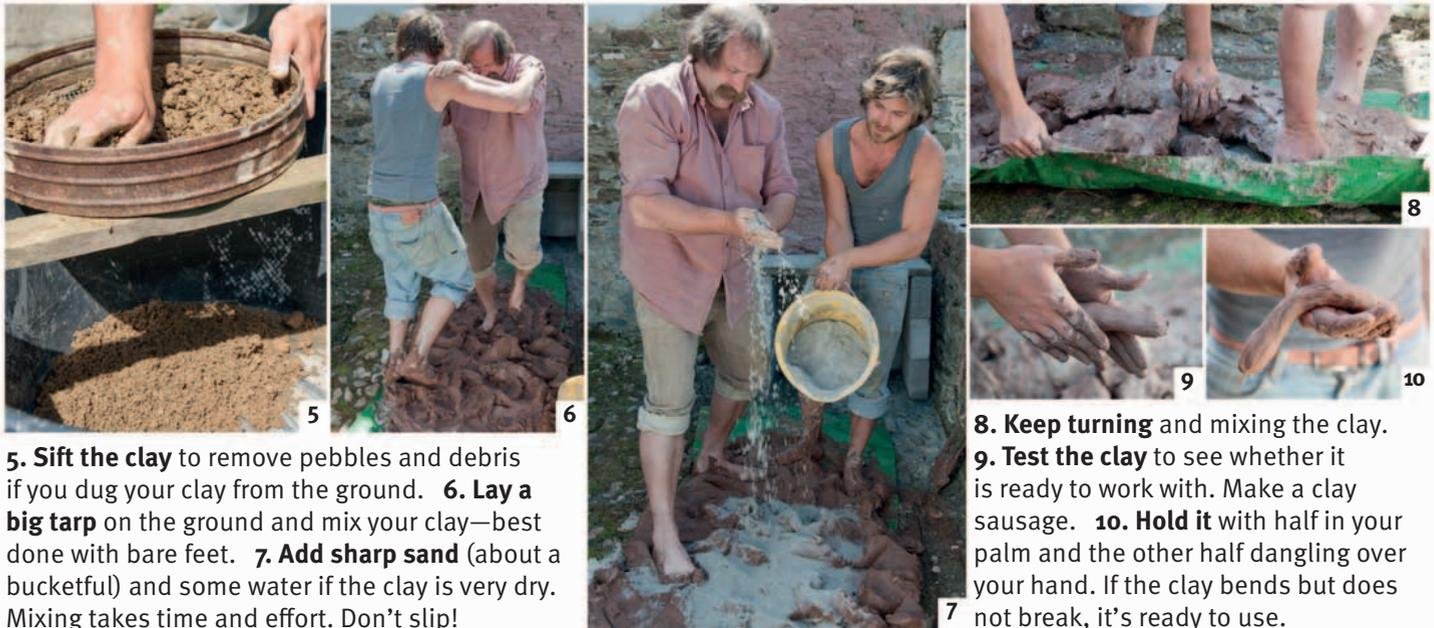
**5. Sift the clay** to remove pebbles and debris if you dug your clay from the ground. **6. Lay a big tarp** on the ground and mix your clay—best done with bare feet. **7. Add sharp sand** (about a bucketful) and some water if the clay is very dry. Mixing takes time and effort. Don't slip!
