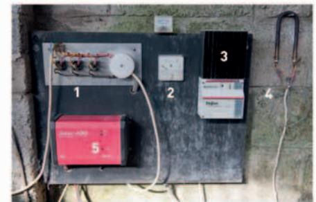
**Converting water energy to electricity** requires the following items: a rectifier (1), ammeter (2), charge controller (3), dump load (4), and pure sine inverter (5).
