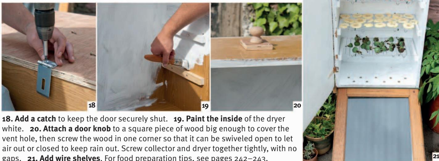
**18. Add a catch** to keep the door securely shut. **19. Paint the inside** of the dryer white. **20. Attach a door knob** to a square piece of wood big enough to cover the vent hole, then screw the wood in one corner so that it can be swiveled open to let air out or closed to keep rain out. Screw collector and dryer together tightly, with no gaps. **21. Add wire shelves.** For food preparation tips, see pages 242–243.
