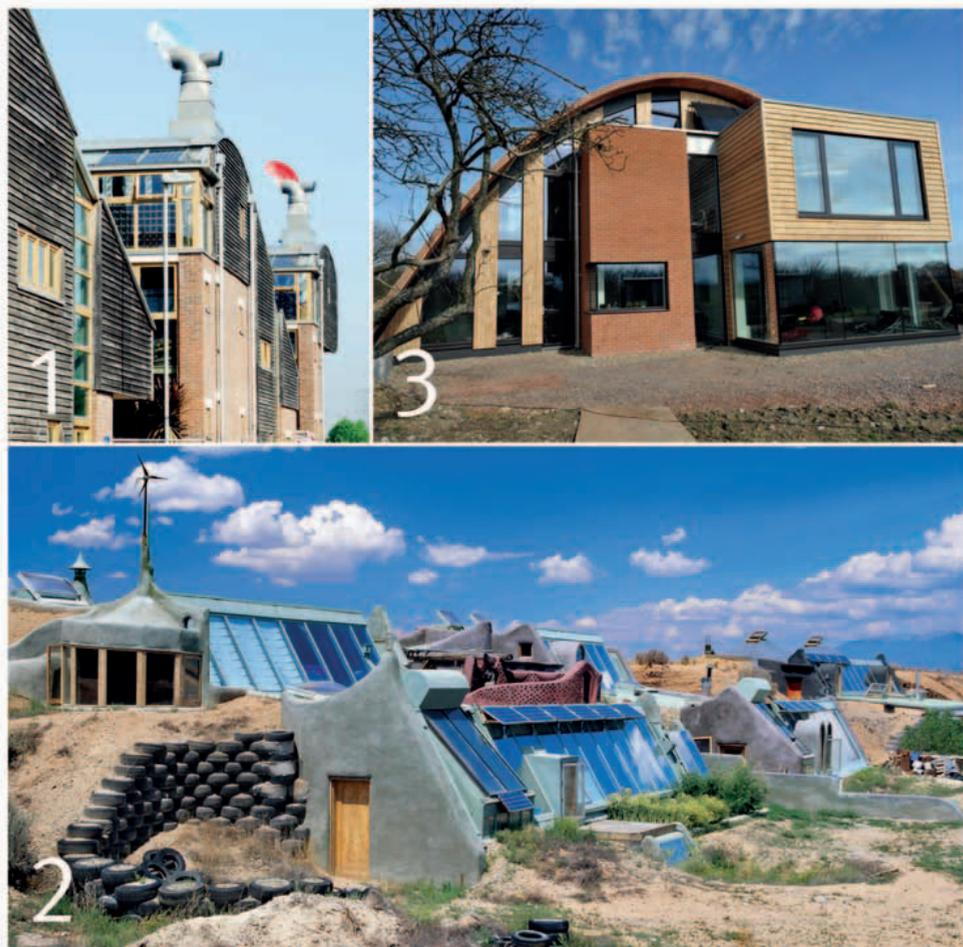
**1. The first environmentally friendly housing development in the UK—Beddington Zero Energy Development (BedZED).** Homes are made from reclaimed or natural materials. **2. Earth shelters in New Mexico** are made from rammed earth and car tires (see pages 48–49). **3. A zero-carbon house in Kent, UK,** needs no fossil fuels for heating. Its vault shape gives it high thermal mass.
