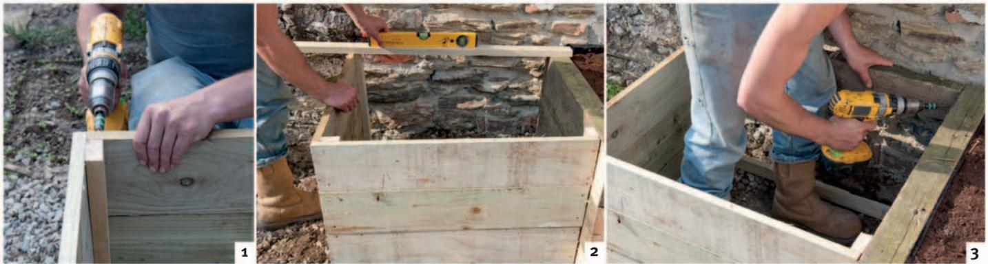
**1. Make a simple box** by screwing horizontal planks to a framework. The size of your box will depend on what you use for a lid. We based ours on an old window. Make the uprights from standard 1 x 2 in (50 x 25 mm) lengths of wood. We used some leftover planks for the sides—1 x 6 in (150 x 25 mm) are ideal—and we saved on wood by positioning the cold frame against a raised bed and wall. **2. Make sure the sides** are level. **3. Add a brace** across the back of the box to keep it square.
