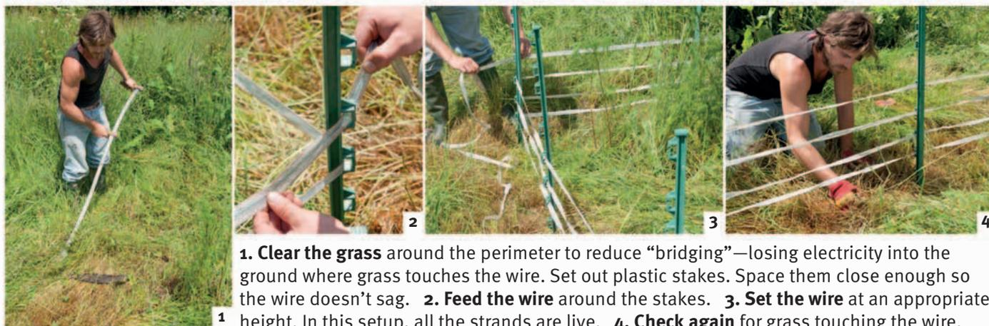
**1. Clear the grass** around the perimeter to reduce “bridging”—losing electricity into the ground where grass touches the wire. Set out plastic stakes. Space them close enough so the wire doesn't sag. **2. Feed the wire** around the stakes. **3. Set the wire** at an appropriate height. In this setup, all the strands are live. **4. Check again** for grass touching the wire.
