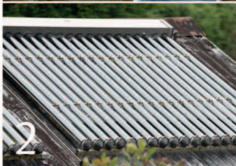
**1.** When we first moved to the farm, there was no plumbing, so we used a camping solar shower. This is a black plastic water carrier that is filled with water and left in full sunlight; within a couple of hours it is hot enough to provide a luxurious shower. **2.** Our solar collectors comprise evacuated tubes with heat pipes connected to the manifold at the top, through which water flows and is heated.
