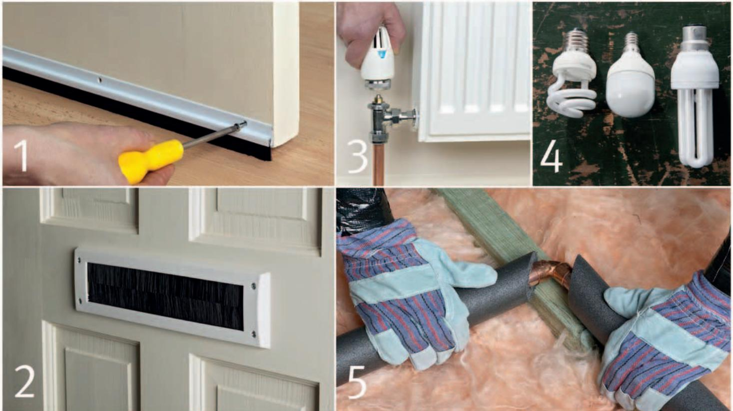
**1. Add door sweeps** to all external doors to keep your home warm. **2. Draft-proof a letterbox** with brush strips. **3. Thermostatic radiator valves** allow you to heat rooms to different temperatures. **4. Low-energy light bulbs** are available in options to suit all fixtures. **5. Insulate pipes** in a cold attic to reduce heat loss.
