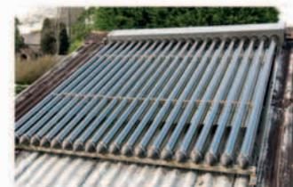
**Solar thermal collectors (13)** warm up water efficiently. Use them to supply a shower in addition with a south-facing roof.
