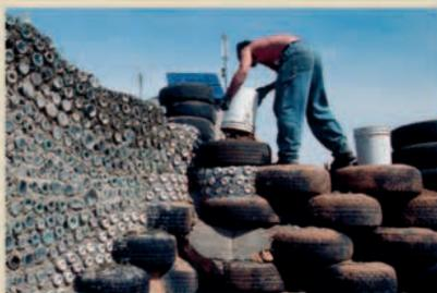
The main part of the structure is built from old car tires (see box left), including a retaining wall for the slope behind and damp-proof course
