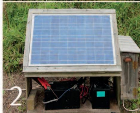
**1. Our grid-linked wind turbine** allows us to sell any excess electricity we create back to the power company. **2. Energy created** by these solar PV panels is stored in deep-cycle batteries for such things as pumping water from our spring.
