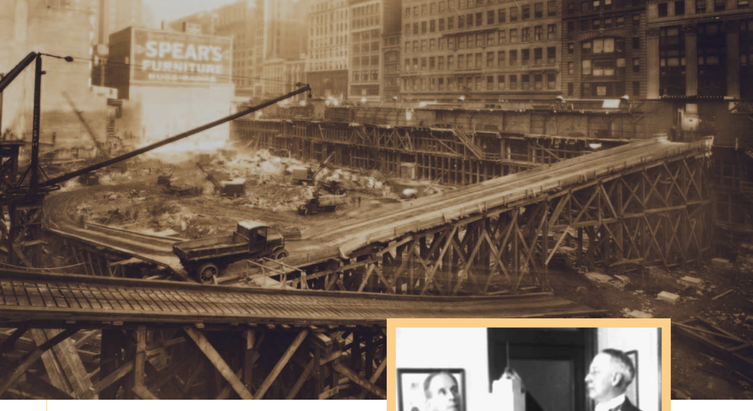
Above: A truck climbs a ramp out of the excavated foundations of the Empire State Building in 1930. Inset: John Raskob (left) and New York governor Alfred Smith (right) examine a model of the Empire State Building.
