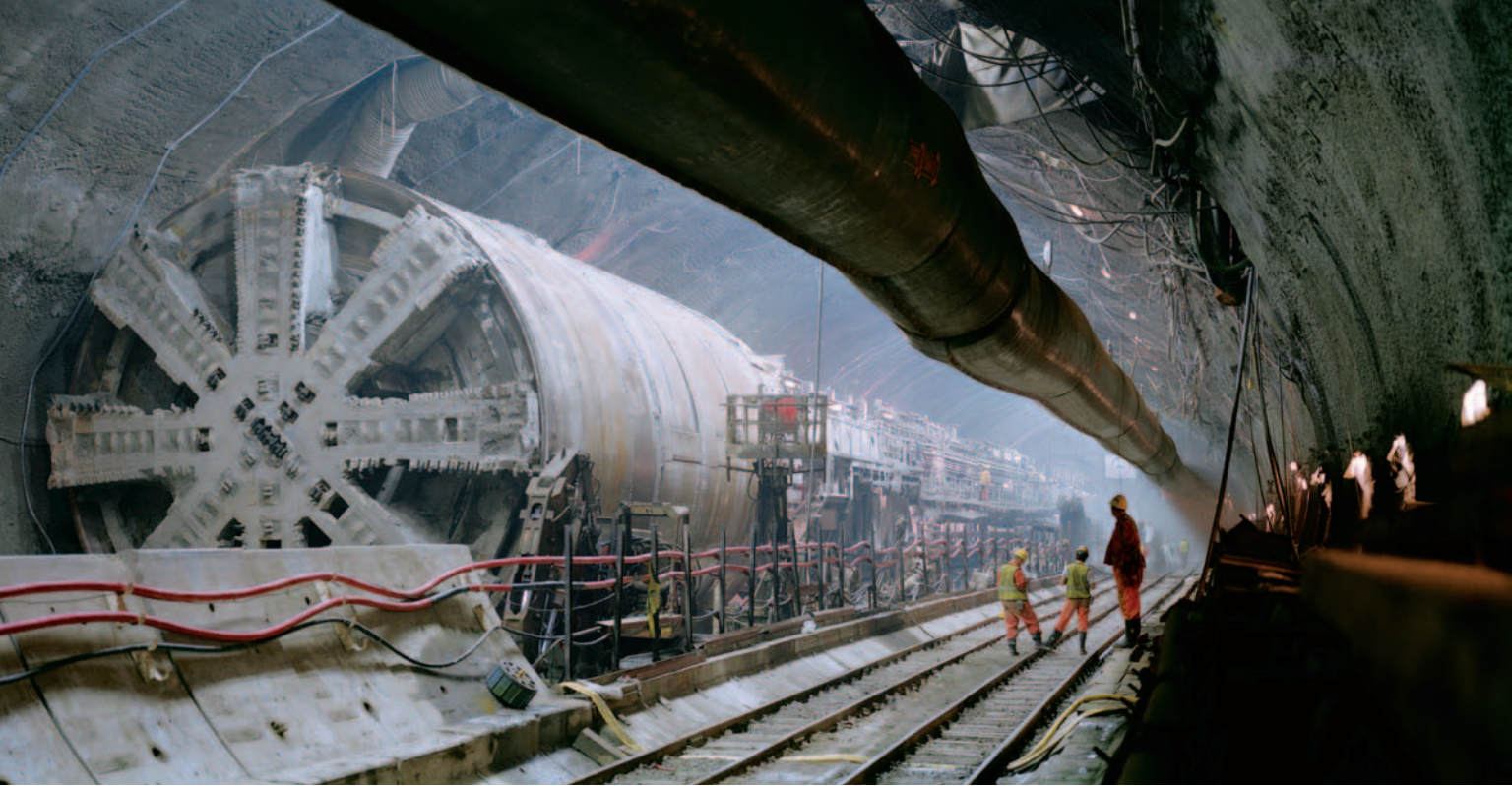
Above: One of the giant tunnel-boring machines moves into position during excavations. Below left: In 1990, French and British engineers make the first breakthrough connecting the tunnel's two ends.
