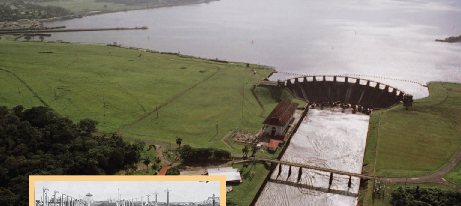
Above: Gatun Dam draws water from the artificial Gatun Lake to control the water level for the Panama Canal. Inset: In 1913 the tugboat Gatun was the first boat to use the Gatun Locks and enter the unfinished canal.
