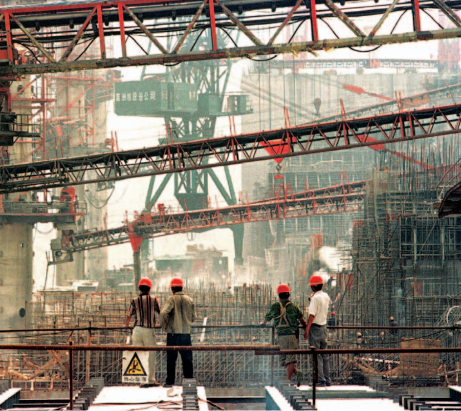
Above left: Workers watch as cranes deliver concrete during construction of the Three Gorges Dam in 2001. Below left: Water gushes out of the dam's power plant. Below right: Cargo ships line up in a lock at the Three Gorges Dam in 2006.
