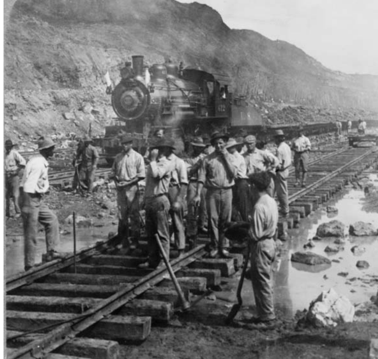
Left: Dynamite crews prepare explosives during the excavation of the Culebra Cut. Right: Workers use shovels to finish excavations after steam shovels dug the main channel of the Culebra Cut.
