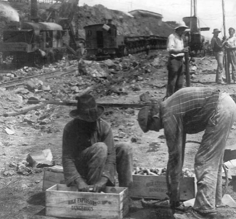
Left: Dynamite crews prepare explosives during the excavation of the Culebra Cut. Right: Workers use shovels to finish excavations after steam shovels dug the main channel of the Culebra Cut.
