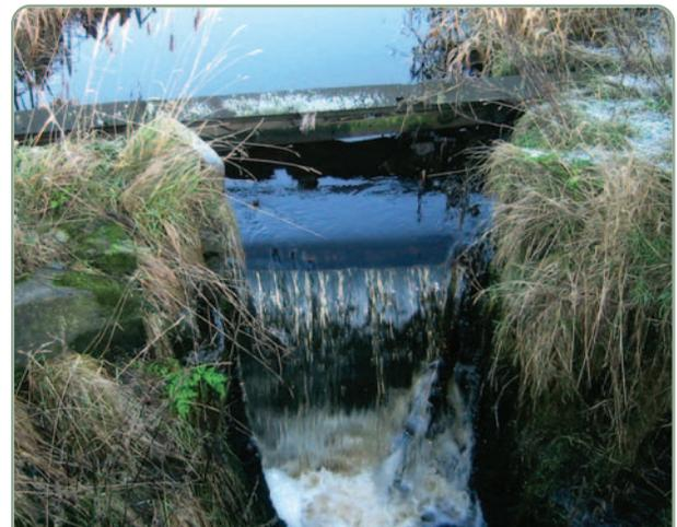
**The weir is a traditional means of microgeneration for projects near to rivers**
