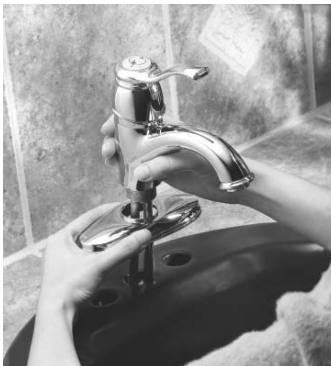
Figure 16.7 Assembling a faucet. Courtesy of Moen, Inc.
