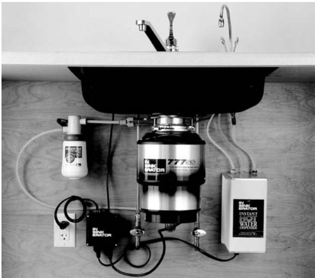
Figure 16.7 Typical garbage disposer installation with hot water dispenser. Courtesy of In-Sink-Erator
